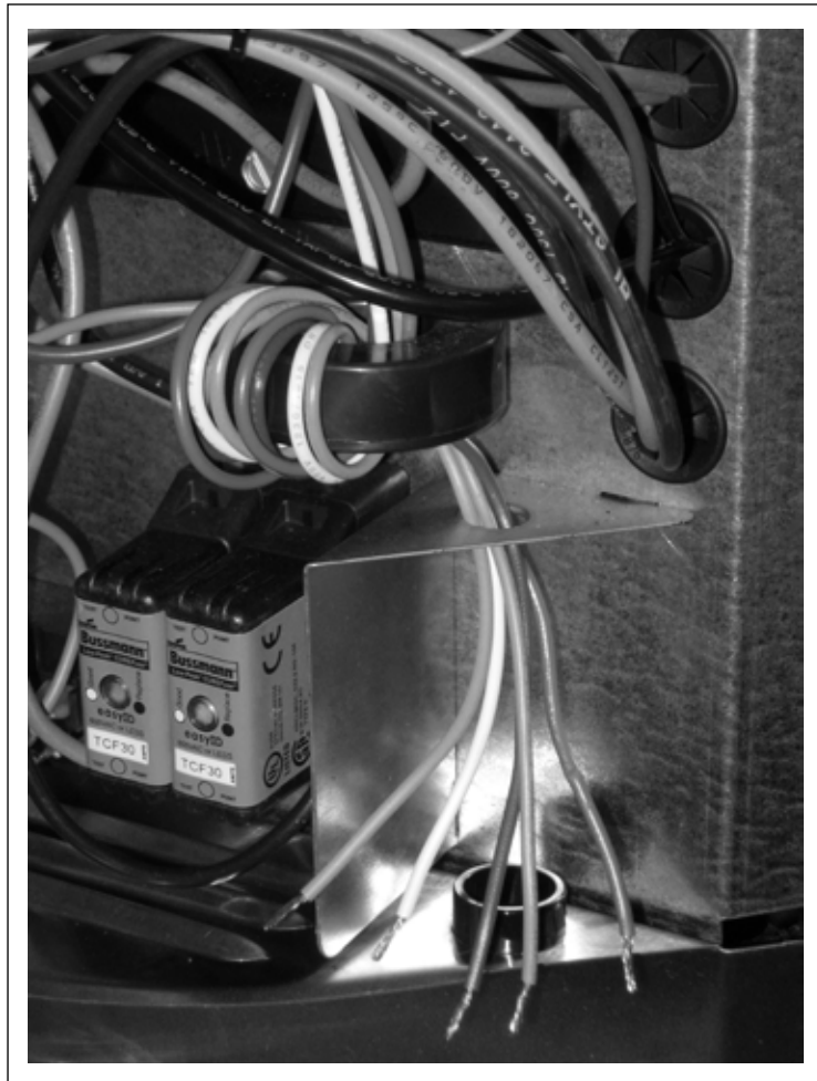
Figure 5. Low Voltage Control Wiring Compartment
